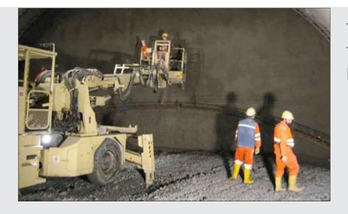
To establish and fix the tunnel arch the customer used a rope and two people baskets.
